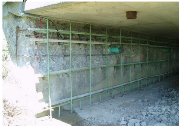
Figure 3 Galvanic Anodes Installed Across the Face of Abutment
