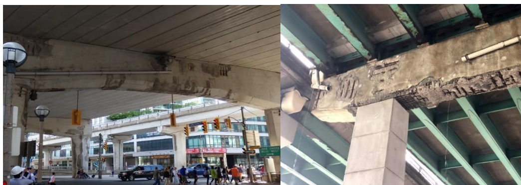
Figure 15, 16 Condition of Structural Elements Prior to Rehabilitation
