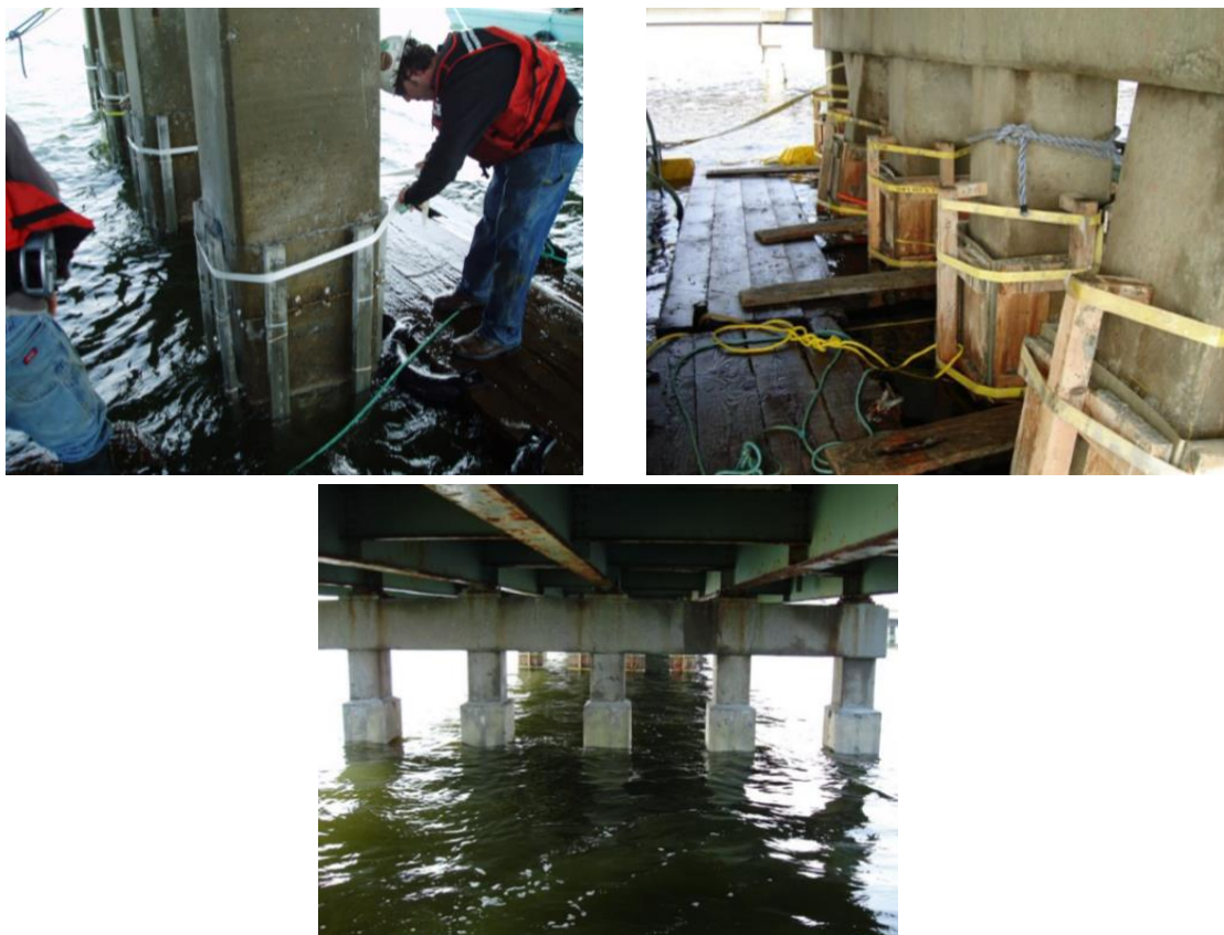
Figures 6, 7, 8 Anode installation, Temporary support of jackets during concrete placement, Completed galvanic pile jackets.
