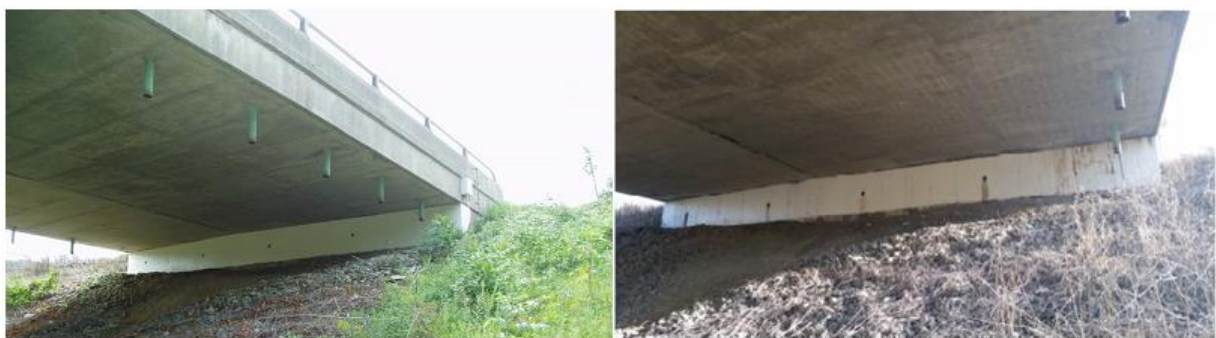
Figure 5 Photos of completed abutment in 2005 and 2020
