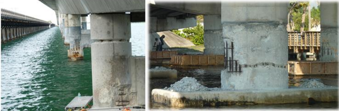
Figure 9 Deteriorated Columns (left) and Damaged Concrete Removed (right)
