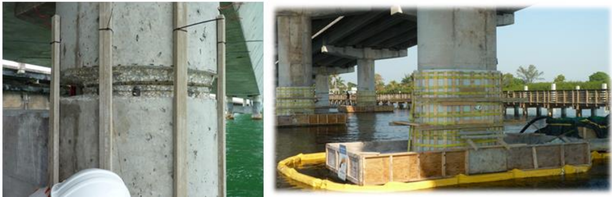
Figure 10 Installation of Alkali-Activated Galvanic Anodes (left) and Stay-in-Place Form Installed (right)
