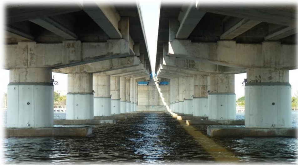
Figure 12 Above-Water Alkali-Activated Galvanic Cathodic Protection Jackets
