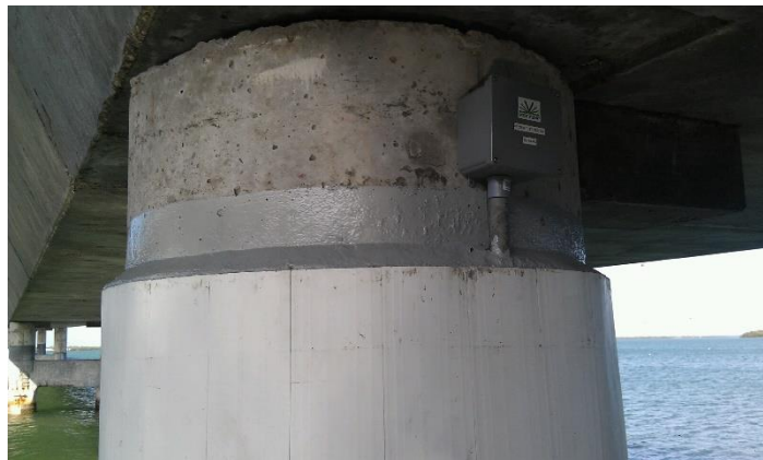
Figure 11 Installed PVC Galvanic Cathodic Protection Jacket with Monitoring Station
